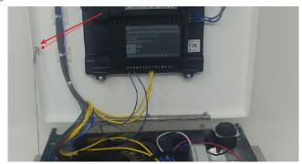
Plug wired connectors from terminal blocks into appropriate input blocks in PLC.
