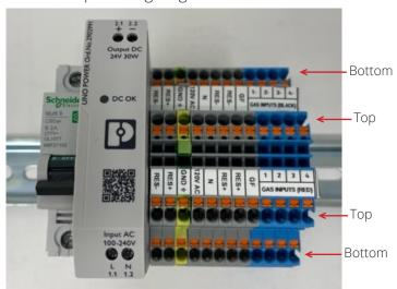
NOTE: The top row of all input terminal blocks (gas inputs and digital signal inputs) is always 24 VDC common. When wiring in gas transducers, the RED wire is always wired into the open input location on the TOP row; the BLACK wire is always wired into the open input location on the BOTTOM row. When wiring digital input signals, the POSITIVE wire is always wired into the open input location on the TOP row; the SIGNAL wire is always wired into the BOTTOM row.
